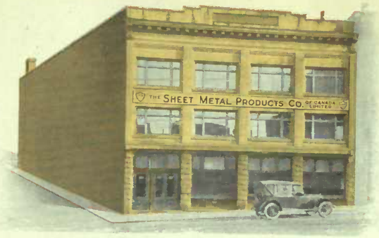
Vancouver Office and Warehouse, Beatty Street, Vancouver.
